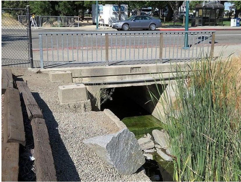
Culvert Under a Road
