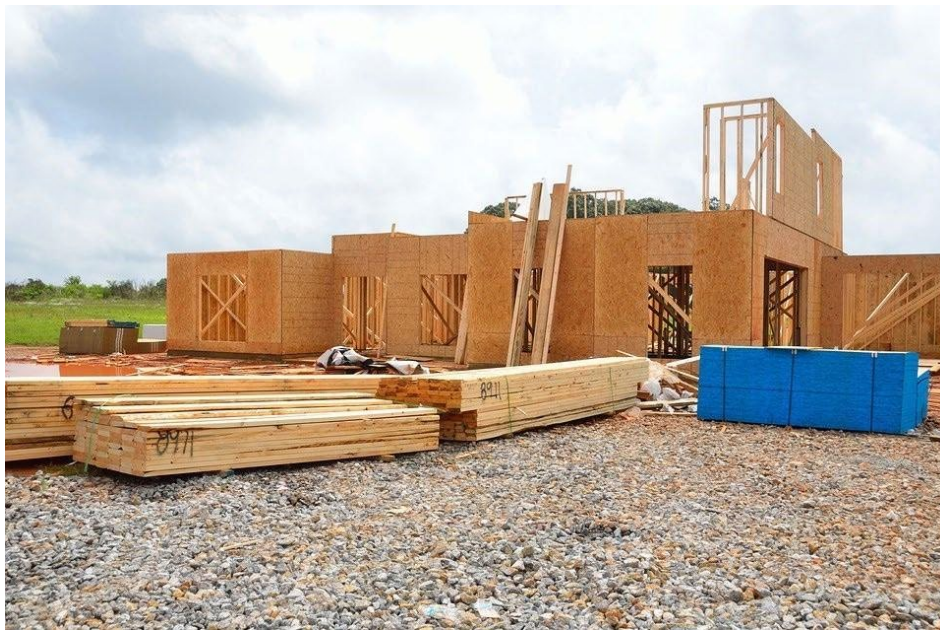
A Wooden Building Under Construction
