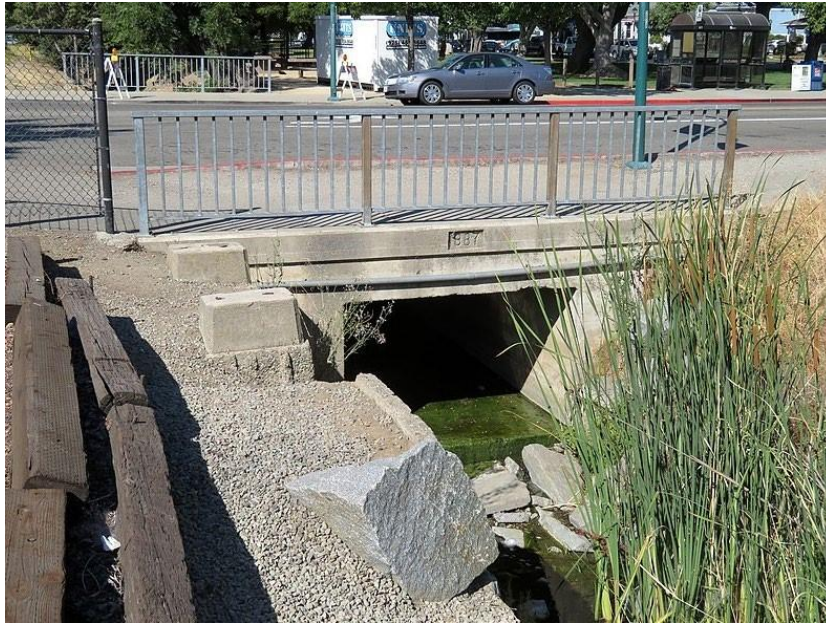
Culvert Under a Road
