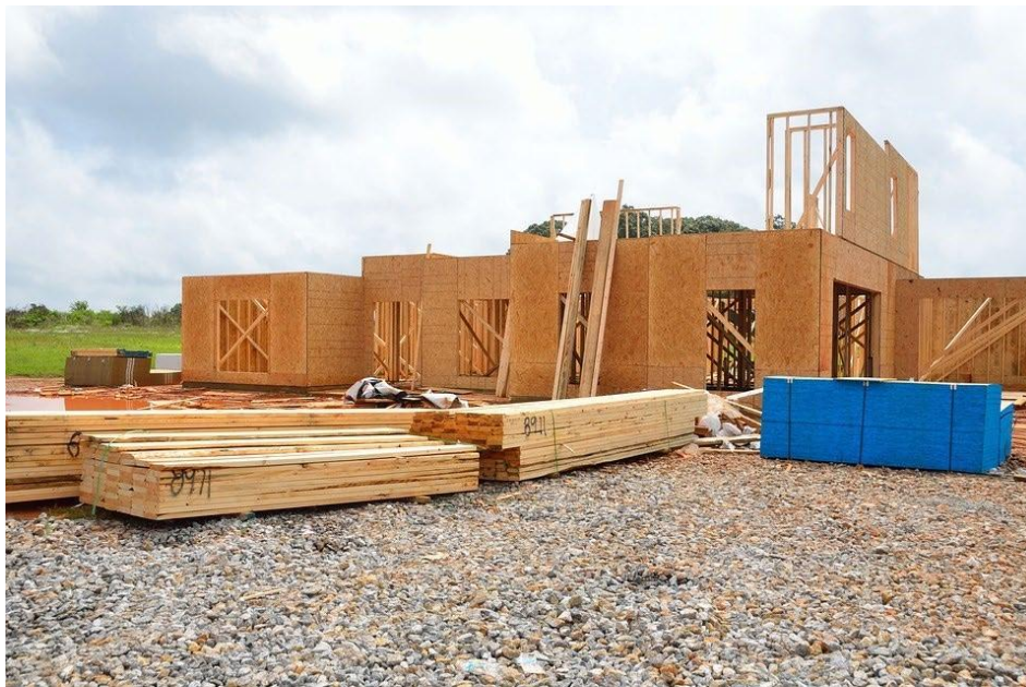
A Wooden Building Under Construction
